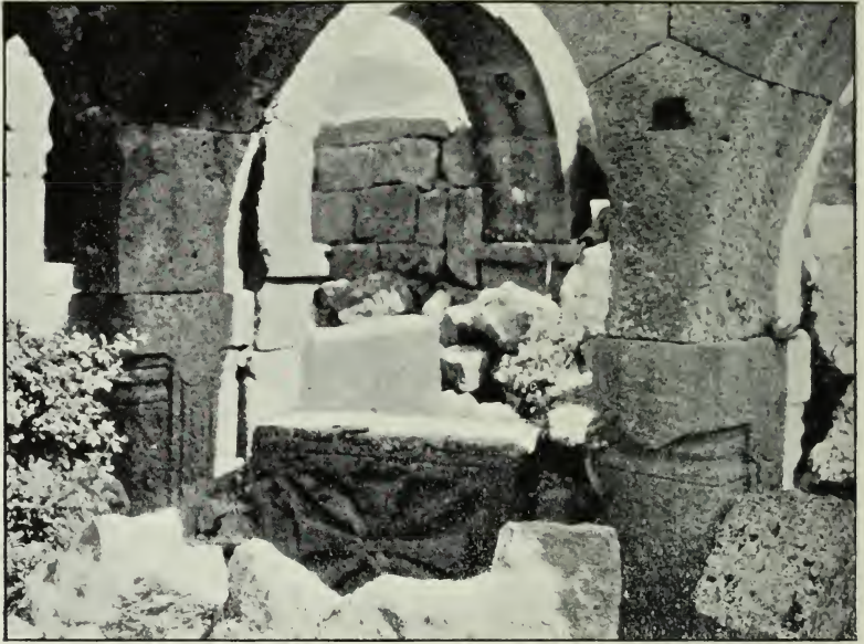
FIG. 124.—No. 31, slab between nave and S. aisle.
